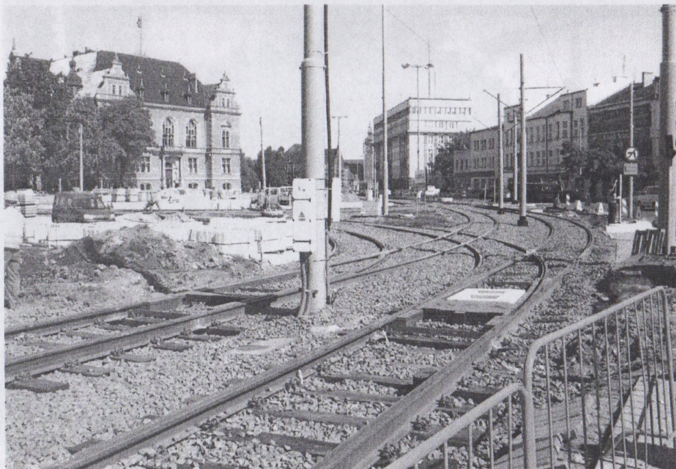
Track reconstruction outside Central Station
